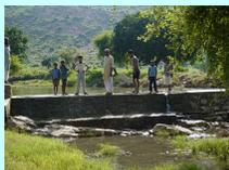
"Check-dams" are small barriers built across the direction of water flow on shallow rivers and streams for the purpose of water harvesting. The small dams retain excess water flow during monsoon rains in a small catchment area behind the structure. Pressure created in the catchment area helps force the impounded water into the ground. Pics- Tarun Bharat Sangh (top), Sehgal Foundation in Haryana (Below)
